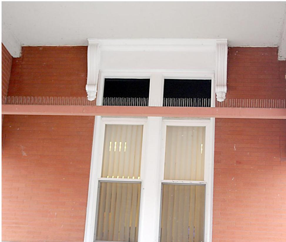
The Inter-Mountain photo by Amanda Hayes Pigeon spike strips like these located under the walkway that connects the Upshur County Courthouse to the annex will be installed around the dome and cupola as part of a plan to discourage pigeons from damaging the structure.
